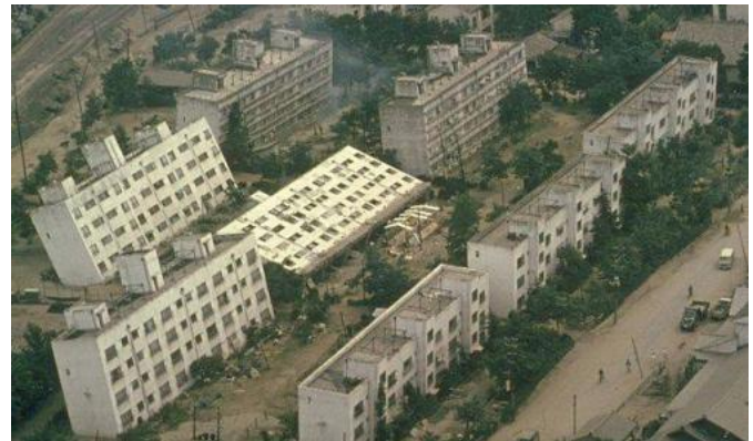
Buildings toppled from liquefaction during a 7.5 magnitude earthquake in Japan.
