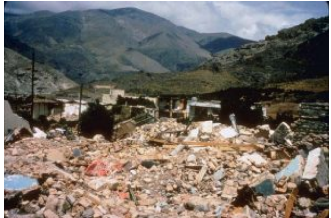
Example of devastation on unreinforced masonry by seismic motion.
