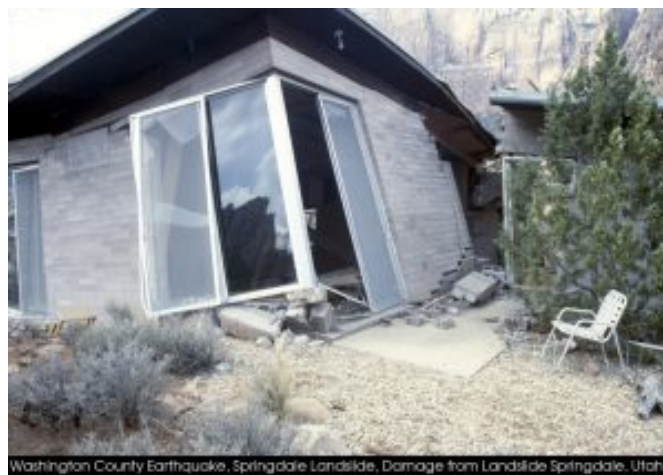
House in Springdale, Utah destroyed by earthquake-triggered landslide.
